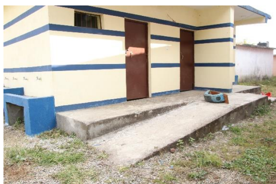
Wheelchair ramp slope in newly constructed toilet found not wheelchair friendly
