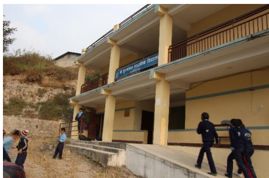
Wheelchair ramp slope in school for the access to PwDs to classroom constructed as per national standards and guidelines
