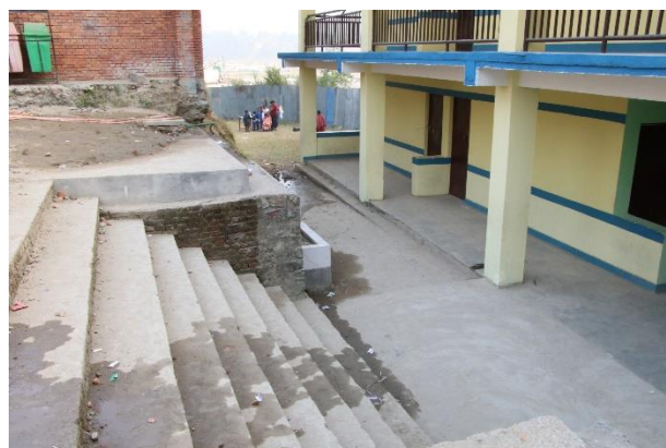
Ladder for the access to classroom in school which is not disabled friendly
